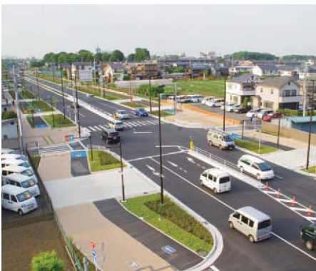
Maintenance of primary local roads (removal of utility poles, promote barrier-free)
