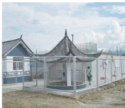
Planning/construction of rural wastewater treatment facilities (China)
