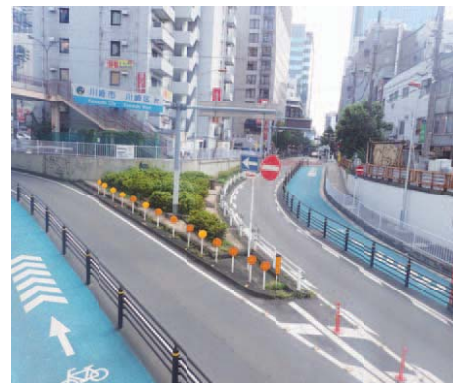
Installation of bicycle lanes in front of stations
