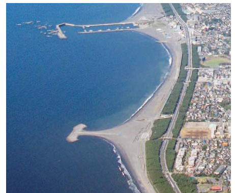
The Headland Plan in the Chigasaki area of Shonan beach (Kanagawa prefecture)
