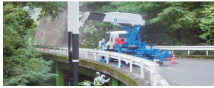
Inspection/diagnosis by bridge inspection vehicles
